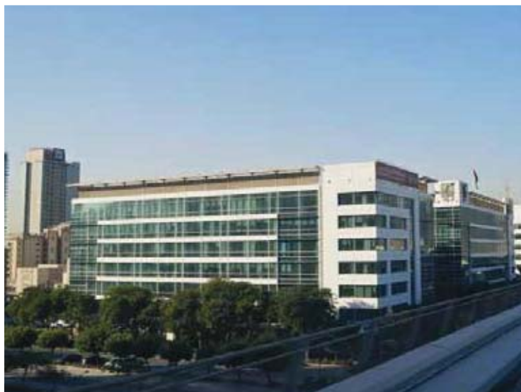
EMAAR BUSINESS PARK BUILDING 4
