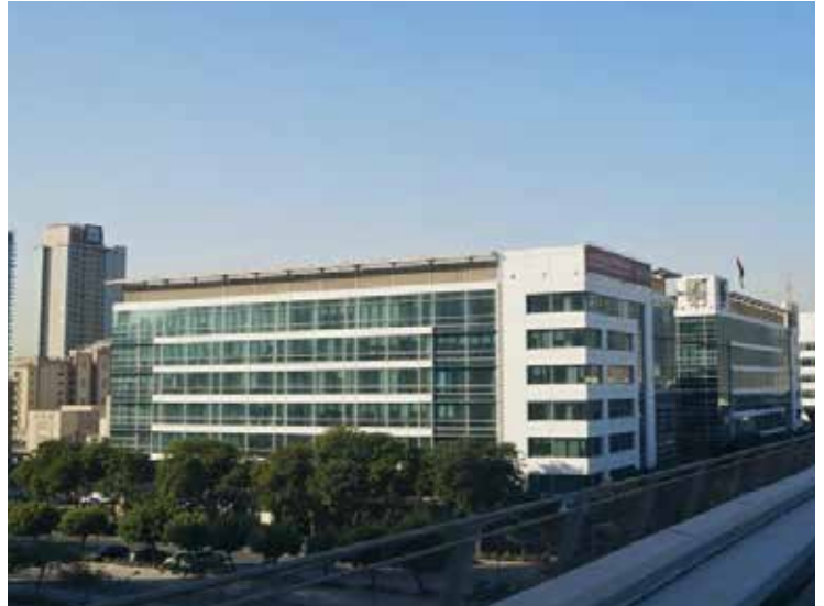
EMAAR BUSINESS PARK BUILDING 4
