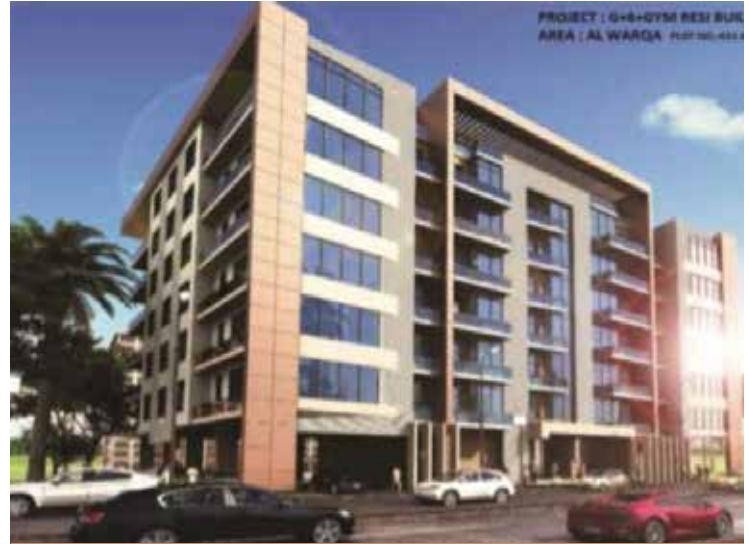
G+6+ RESI BUILDING - AL WARQA
