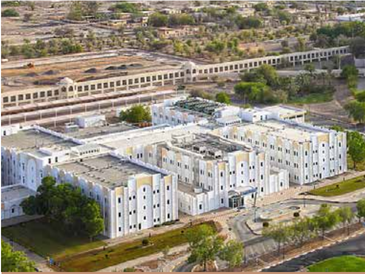
TAWAM HOSPITAL AL AIN (VIP) ROOMS (PHASE ONE)
