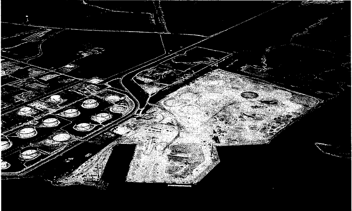
(Picture taken at onset of project in March 2019. )
