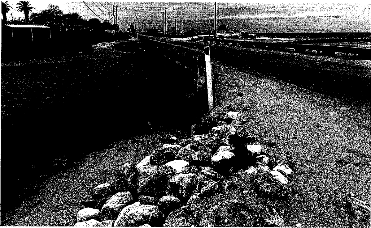
Figure 3. Site photo of Magnolia inlet at Ocean Drive.
