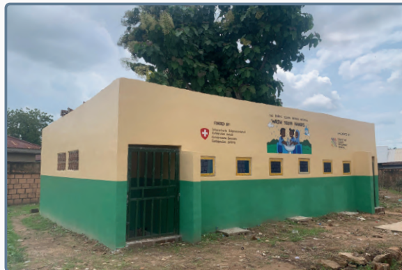
After: The renovated structure!
