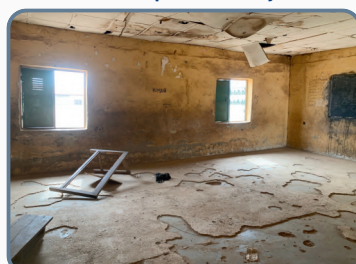
The state of the classroom before renovations at LEA Primary School, Kabusa, Abuja.
