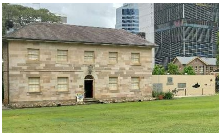
Figure 3.3 Lancer Barracks' Parade Ground and Memorial, Parramatta, NSW
