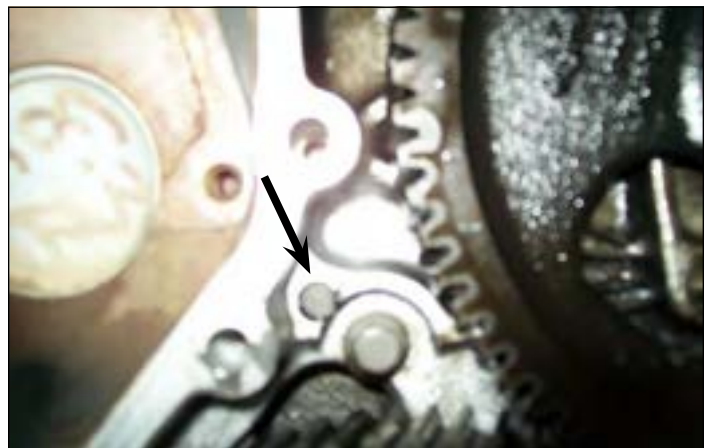
The loose dowel pin on Joe's First Generation truck. The dowel pin have moved out about a quarter of an inch meaning it is ready to fall out.
