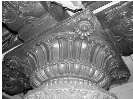
The view of stambha capital with nagas supporting the square plate at Sri Mallikarjuna temple at Canacona
