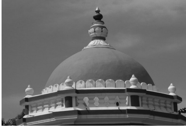
Stupi --- dome on Hindu temples with Anda of stupa surrounded by railings and kalasha replacing the harmika
