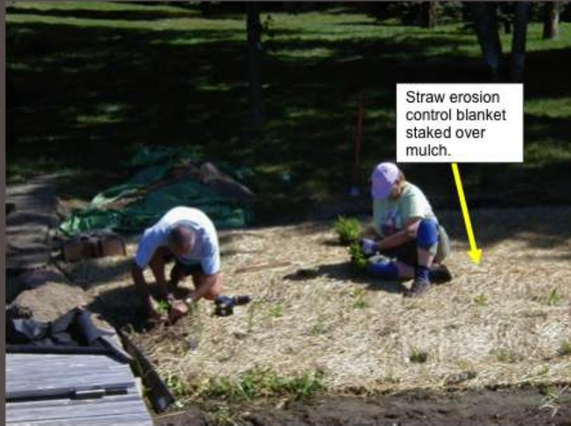
If high water or flooding is possible, a straw erosion control blanket is staked over the mulch prior to planting to prevent the mulch from being washed out. The blanket should have bio-degradable netting. Synthetic photo degradable netting often lasts many years and animals can get caught in the netting.
