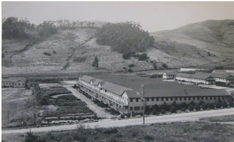
A view of the Sharp Park internment camp (today the archery range) during World War II.
