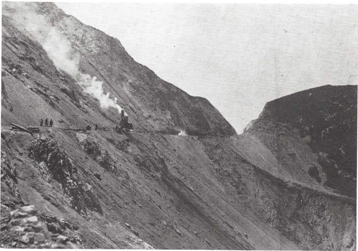
Steam shovel working on slide at Pedro Point
