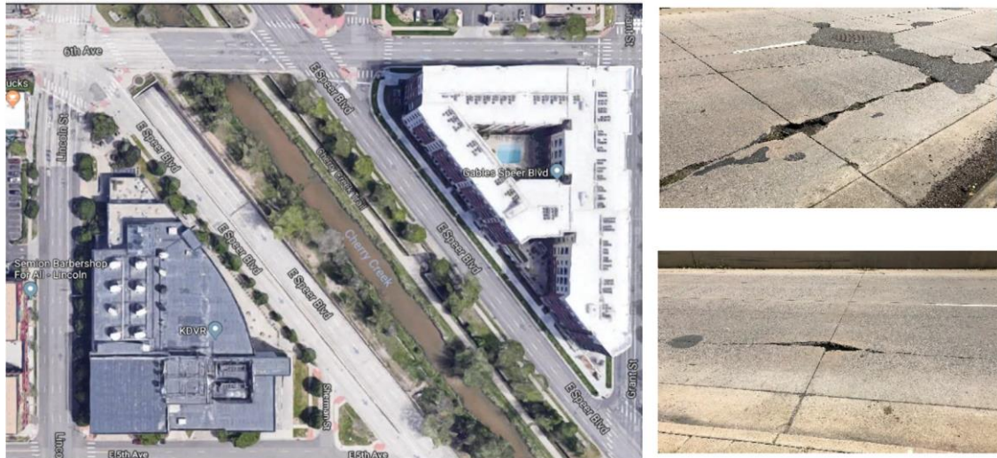
Fig. 2. Site location and condition of concrete pavement to be replaced by City and County of Denver Maintenance Department (M. M. Patel et al. 2016).
