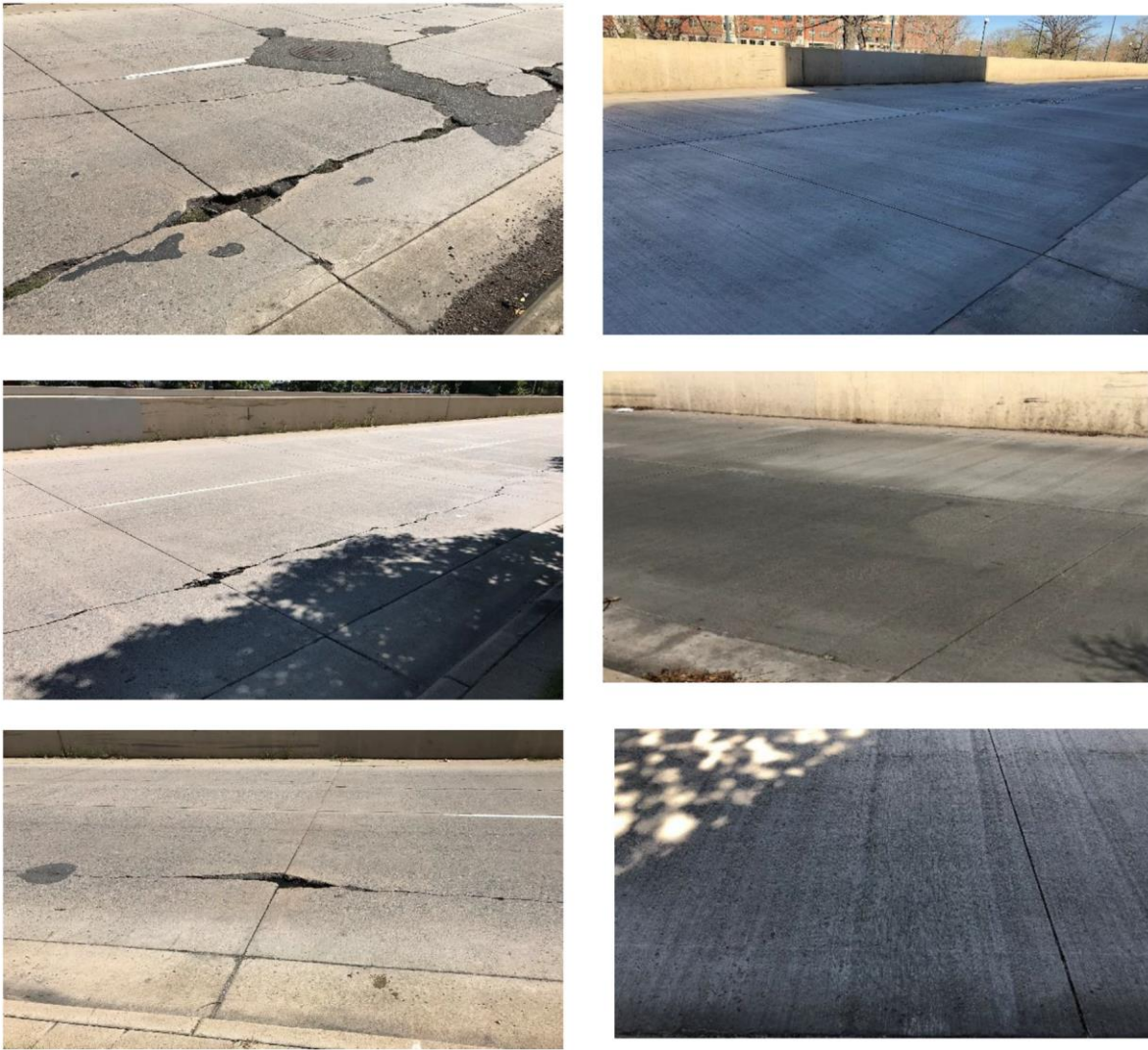
Fig. 5. Field observations of test mixes: Reference mix after five years (left), sample mixes after six months, and one winter (right).
