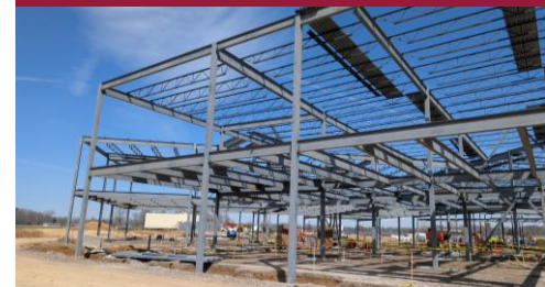
Steel framing at a classroom wing
