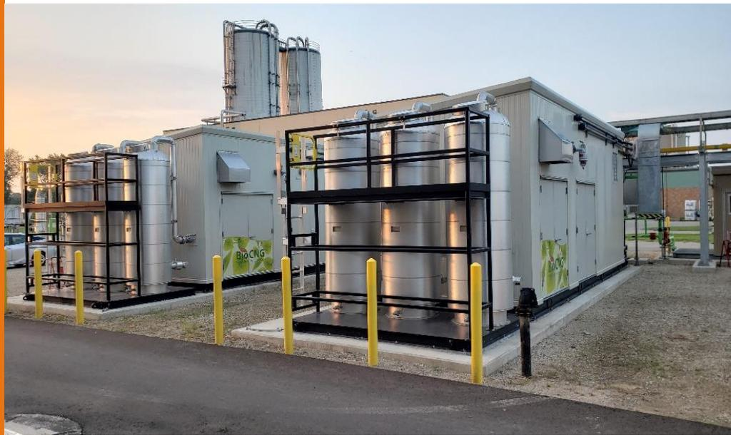
Moisture, bacteria, CO<sub>2</sub> and siloxane/VOC removal
