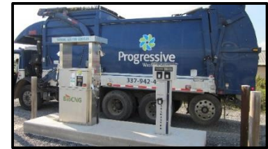
CNG Vehicle Fueling Station
