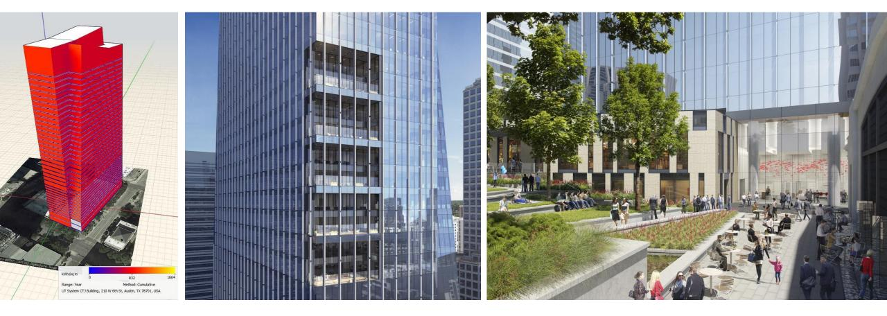
**Intention** High performance glazing & vertical fins to reduce peak heat gain. Efficient mechanical, electrical, plumbing.
