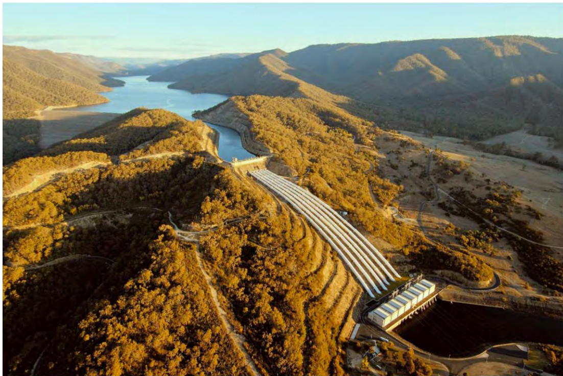
Figure 5: Tumut 3 Power Station, which is within an on-river hydroelectric scheme, image from [11]
