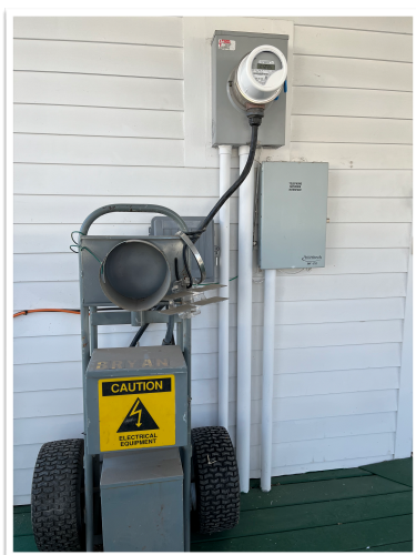
Xcel Energy to the rescue: a problem with current flow. Temporary transformer.
