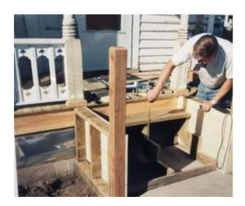
Then the structure for the staircase, including the inside trim boards and their design to echo the design in the spindles of the railing surrounding the entry porch.
