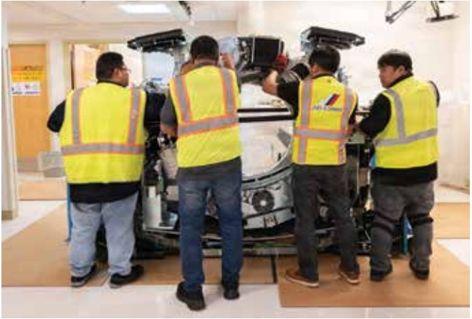
Workers at U.S. Naval Hospital Guam (USNH Guam) install a new Revolution Ascend Plus 72 kilowatt computed tomography (CT) scanner, Feb. 13. Photo credit Hospital Corpsman First Class Clie Lester Guico U.S. Navy
