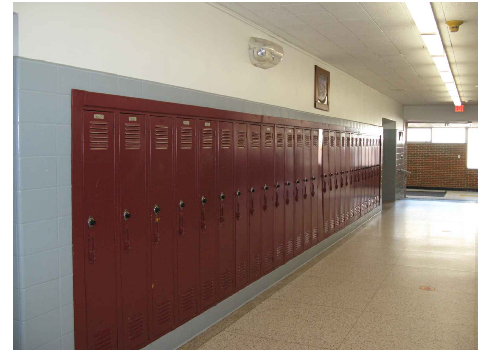
P2 PHOTO: TYP. LOCKER BANK SCALE: NTS PROTECT TILE WAINSCOT & LOCKERS, PATCH & REPAINT PLASTER ABOVE.
