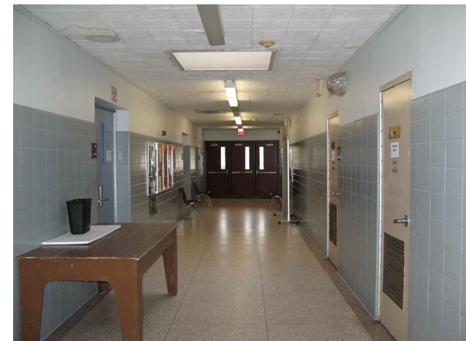
P3 PHOTO: CORRIDOR NW SCALE: NTS TYPICAL CONDITIONS WITHOUT LOCKERS OR DISPLAY CASES. PLASTER WALL FINISHES ARE APPLIED TO TERRA COTTA PARTITION BLOCKS.
