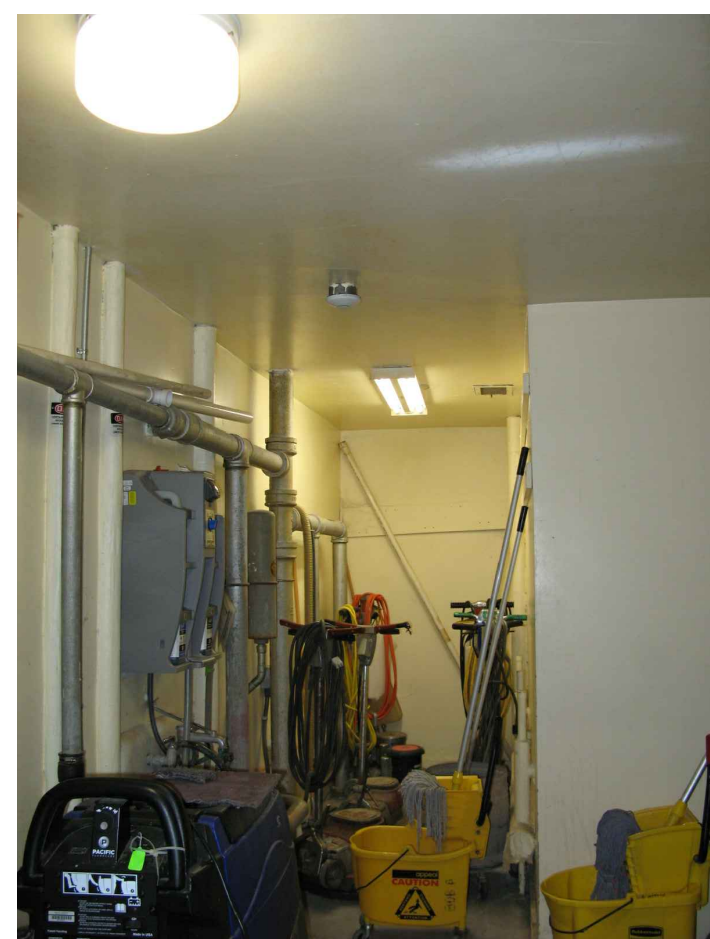
PHOTO: J.C. 24 PIPE CHASE SCALE: NTS NOTE: PLASTER WALL & CEILING PATCHING SHALL BE REQUIRED THIS AREA. REPAINT AREAS PATCHED.
