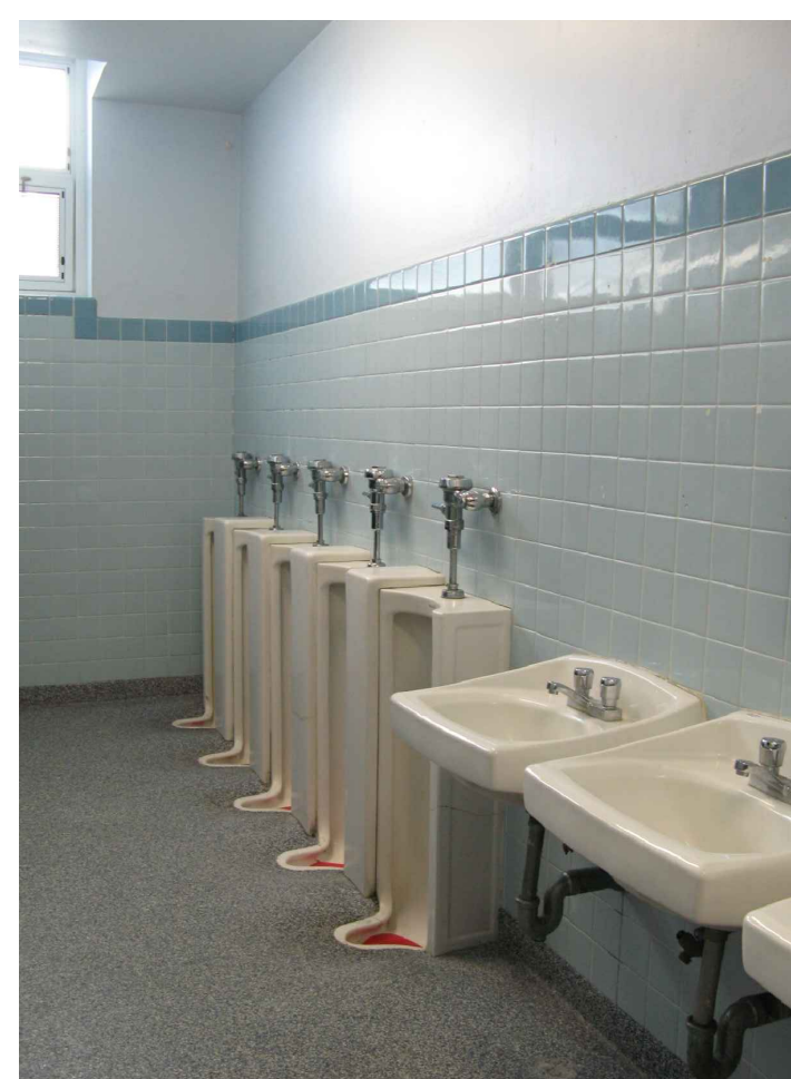
P10 PHOTO: BOYS RESTROOM 26 SCALE: NTS PROTECT TILE WAINSCOTING, TOILET PARTITIONS, AND PLUMBING FIXTURES, TYPICAL IN RESTROOMS.
