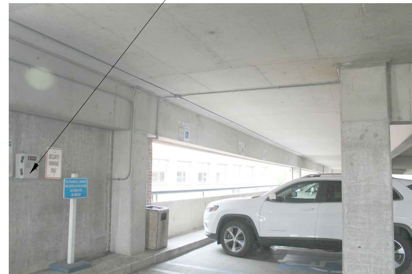
ALL EXISTING CAMERA AND ELECTRICAL FEEDS ARE TO BE RELOCATED TO ALLOW FOR NEW SECURITY BOOTH. CONSTRUCTION CONTRACTOR TO COORDINATE ALL ELECTRICAL, DATA AND CAMERA SERVICE INTERRUPTIONS WITH BUILDINGS AND GROUNDS PRIOR TO DISCONNECTING. (TYP.)
