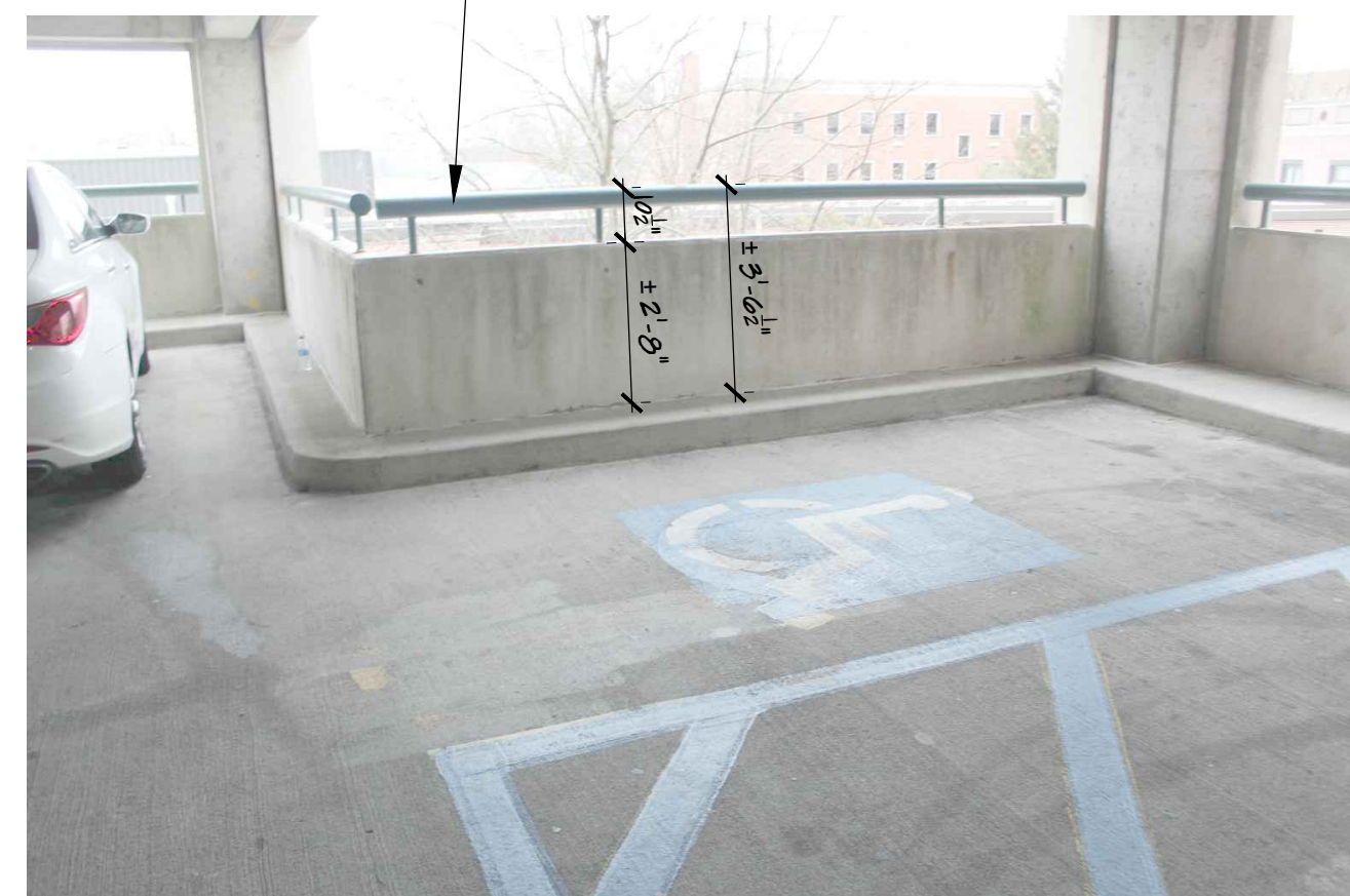
EXISTING RAILING TO BE REMOVED - CONTRACTOR TO PATCH ALL HOLES AND INSTALL NEW PRECAST CONC. SILL - SEE PROPOSED SECTION (TYP.)
