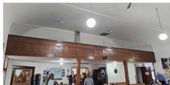
The balcony glass is installed!
