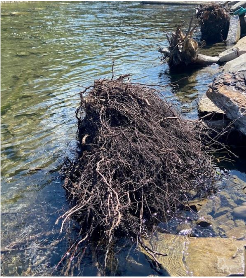
Root wads were placed along the banks at KAG 180 to stabilize them and create fish habitat.
