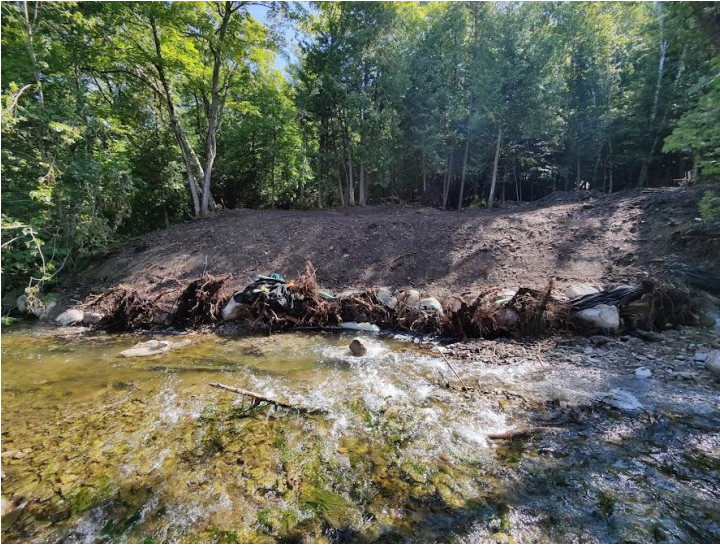
Root wads and boulders were placed along the bank to stabilize it and create habitat for fish. The steep bank was turned into a more gradual slope that was filled with native plants including milkweed for monarchs and pollinators.
