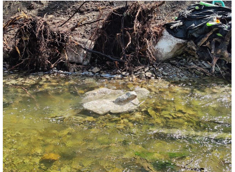
Root wads and boulders were placed along the bank to stabilize it and create habitat for fish. The steep bank was turned into a more gradual slope that was filled with native plants including milkweed for monarchs and pollinators.
