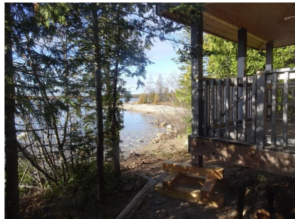
New location, 40 ft. back from water
