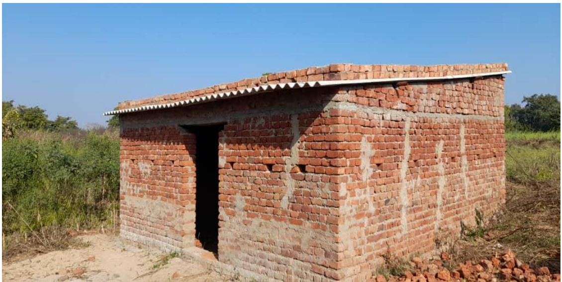
Picture: A newly built house with sheet roof instead of concrete roof in Sinjo
