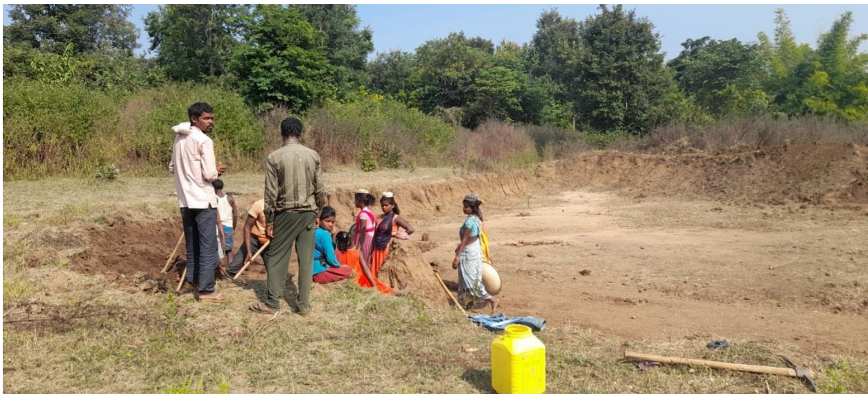
Picture: MGNREGA Worksite (DobhaNirman) in Sinjo
