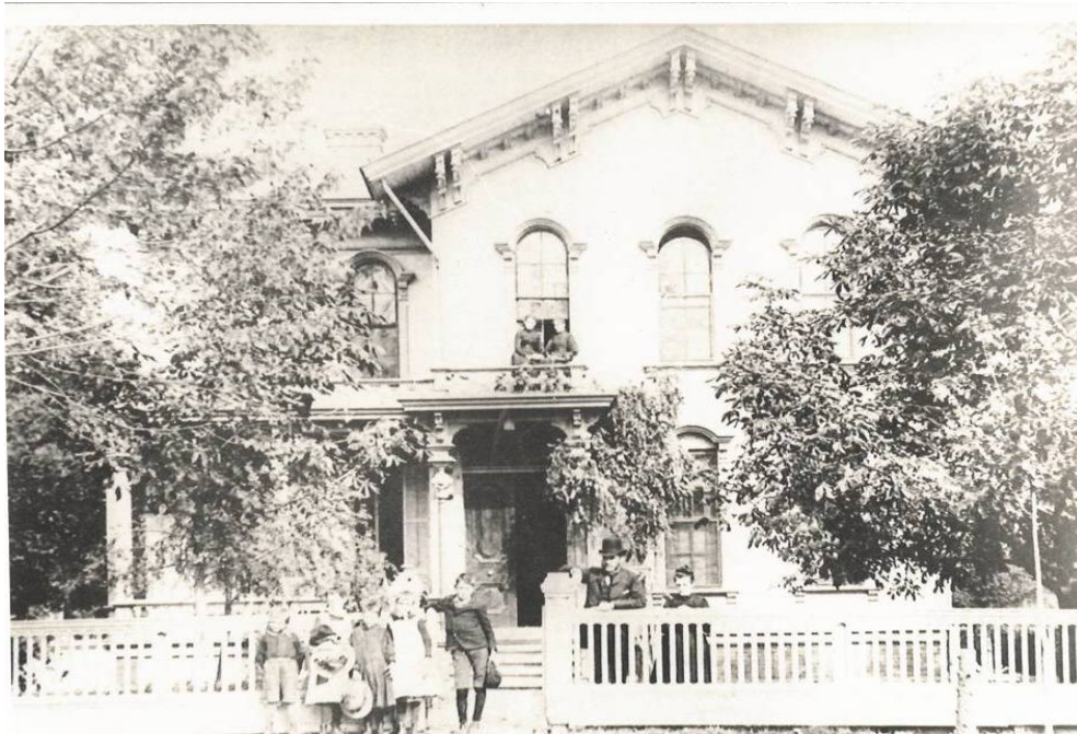
The servants are posed atop the porch in this Crocker family photograph. c. 1881
