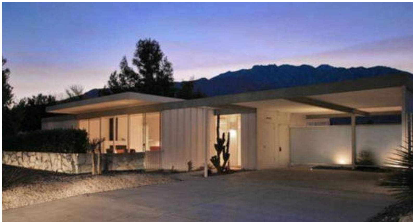
1962 - The Calcor/Rheem Prefabricated Steel House, aka Wexler Steel House 4 of 7, 3133 Sunny View Drive , Palm Springs CA. Commissioned 1961. Developed by the
