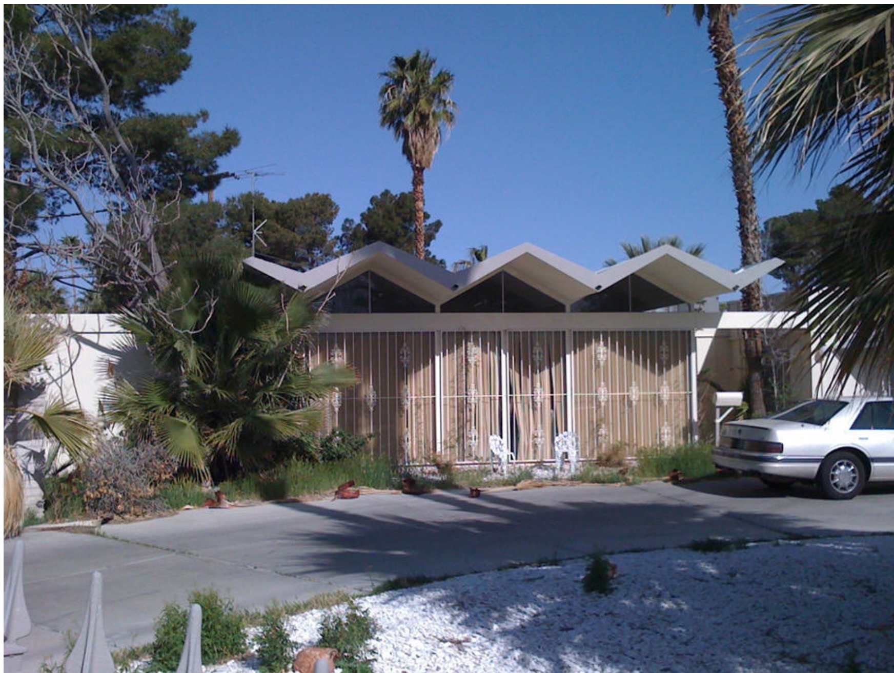
Around 1960 - The Steel House, 1230 Mason Street , Las Vegas NV. Photo by Brad Dunning.
