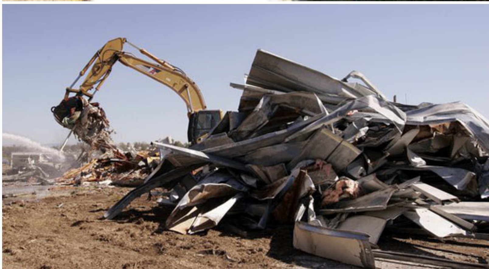
1964 - The Leisure Life Village, 6127 Erlanger Street , San Diego CA. Originally started by architect William Krisel . Builder and developer, Irvin J. Kahn. 248 single story steel apartment homes designed for active adults. Destroyed in 2009 for the 368-unit Cresta Bella Apartments.
