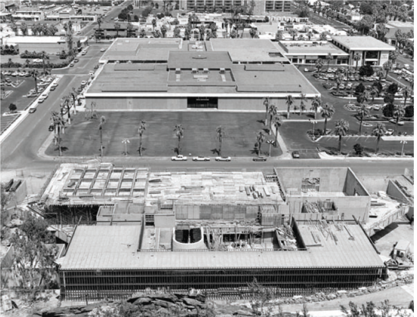
Aerial view of construction in process at Museum Drive, 1970s
