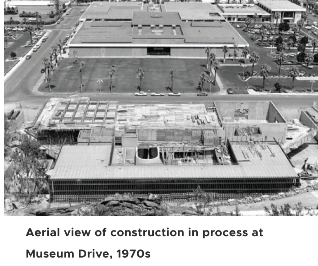
Aerial view of construction in process at Museum Drive, 1970s
