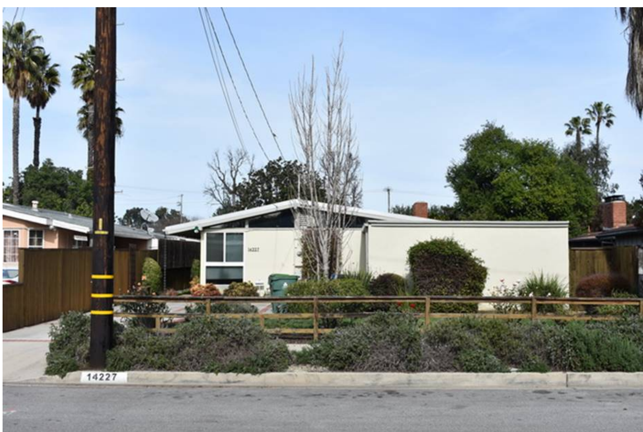
1954 – 14227 West Runnymede Street, Van Nuys CA. Designed with Dan Palmer. Developed by Woodview Homes, Inc., Murray M. Strauss & Assoc., Inc. General Contractors as part of the Modern Gables Tract. Photo by Michael Locke.
