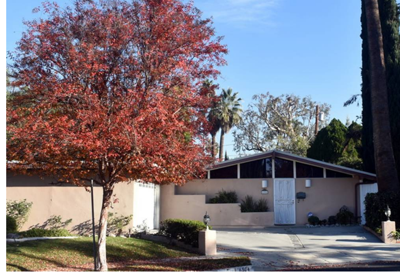
1954 – 6504 Hatillo Avenue, Woodland Hills CA. Designed with Dan Palmer. Developed by the George Alexander Construction Company as part of the Corbin Palms Tract. Photo by Michael Locke.
