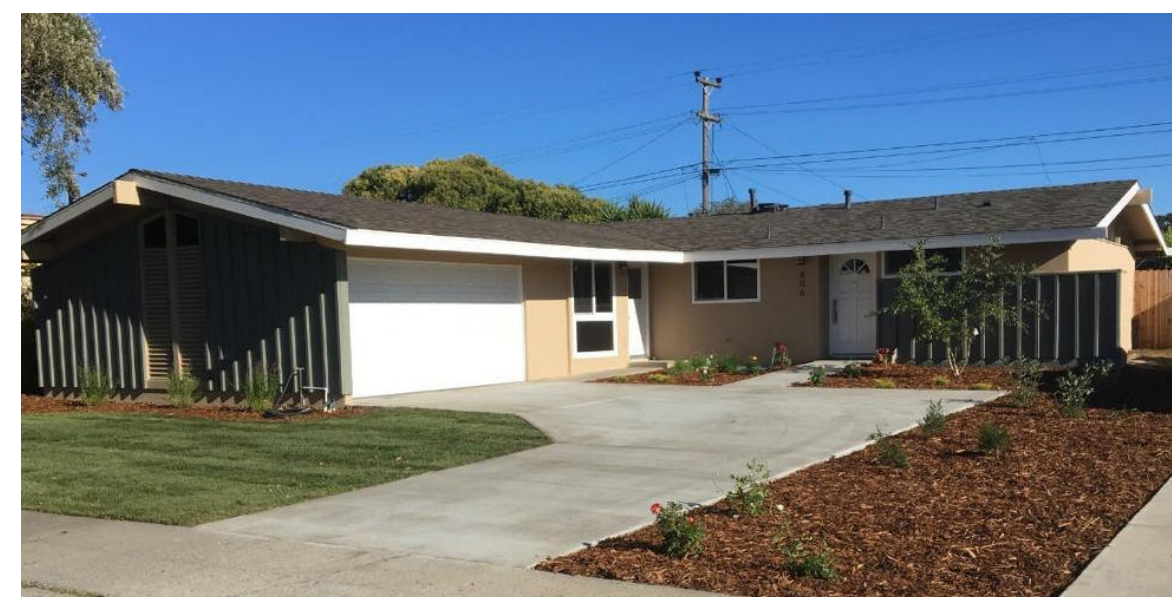
1958 - The Armstrong Homes, Santa Maria CA. Above example is 806 East Tunnell .
