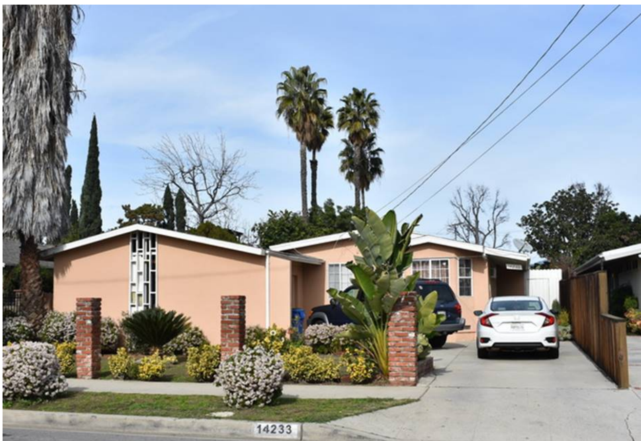
1954 – 14233 West Runnymede Street, Van Nuys CA. Designed with Dan Palmer. Developed by Woodview Homes, Inc., Murray M. Strauss & Assoc., Inc. General Contractors as part of the Modern Gables Tract. Photo by Michael Locke.
