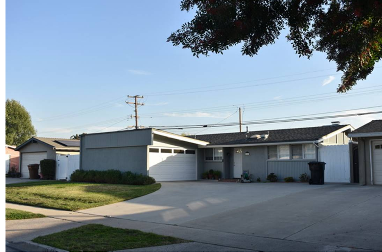
1955 – 2428 Santa Clara Avenue, Fullerton CA. Designed with Dan Palmer. Developed by Midland Properties as part of the Midland Park Estates Subdivision. Photo by Michael Locke.
