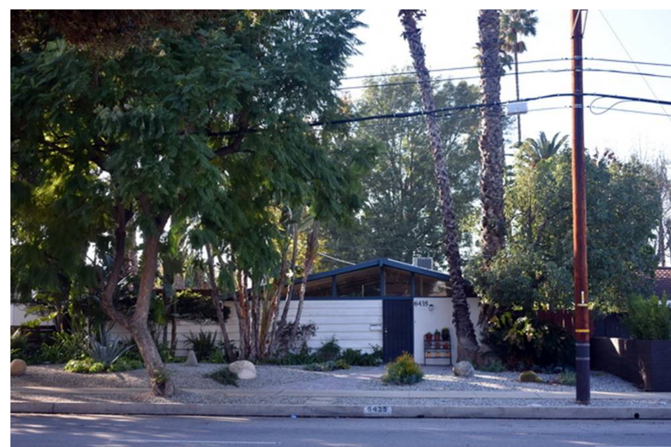
1953 – 6435 Corbin Avenue, Woodland Hills CA. Designed with Dan Palmer. Developed by the George Alexander Construction Company as part of the Corbin Palms Tract. Photo by Michael Locke.
