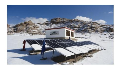
We know that STC operation almost never happens. The array open-circuit voltage was very close to the charge controller rating. We should check to see  $V_{OC,array}(5^{\circ}C) = 3 \times 48.31 \left(1 + \frac{-0.29}{100} \times (5-25)\right)$  if the controller can be used if the if the controller can be used if the temperature is low (why?). Assume the lowest cell temperature will be 5° C. Can the controller be used?
