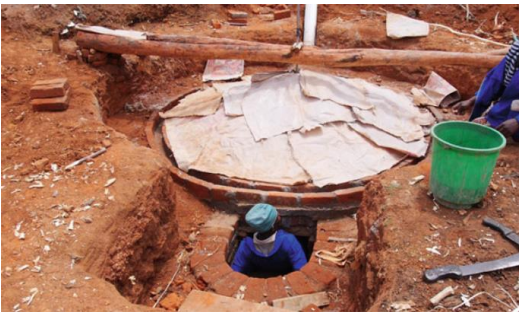
Biogas digester under construction in Malawi (courtesy P. Dauenhauer)
