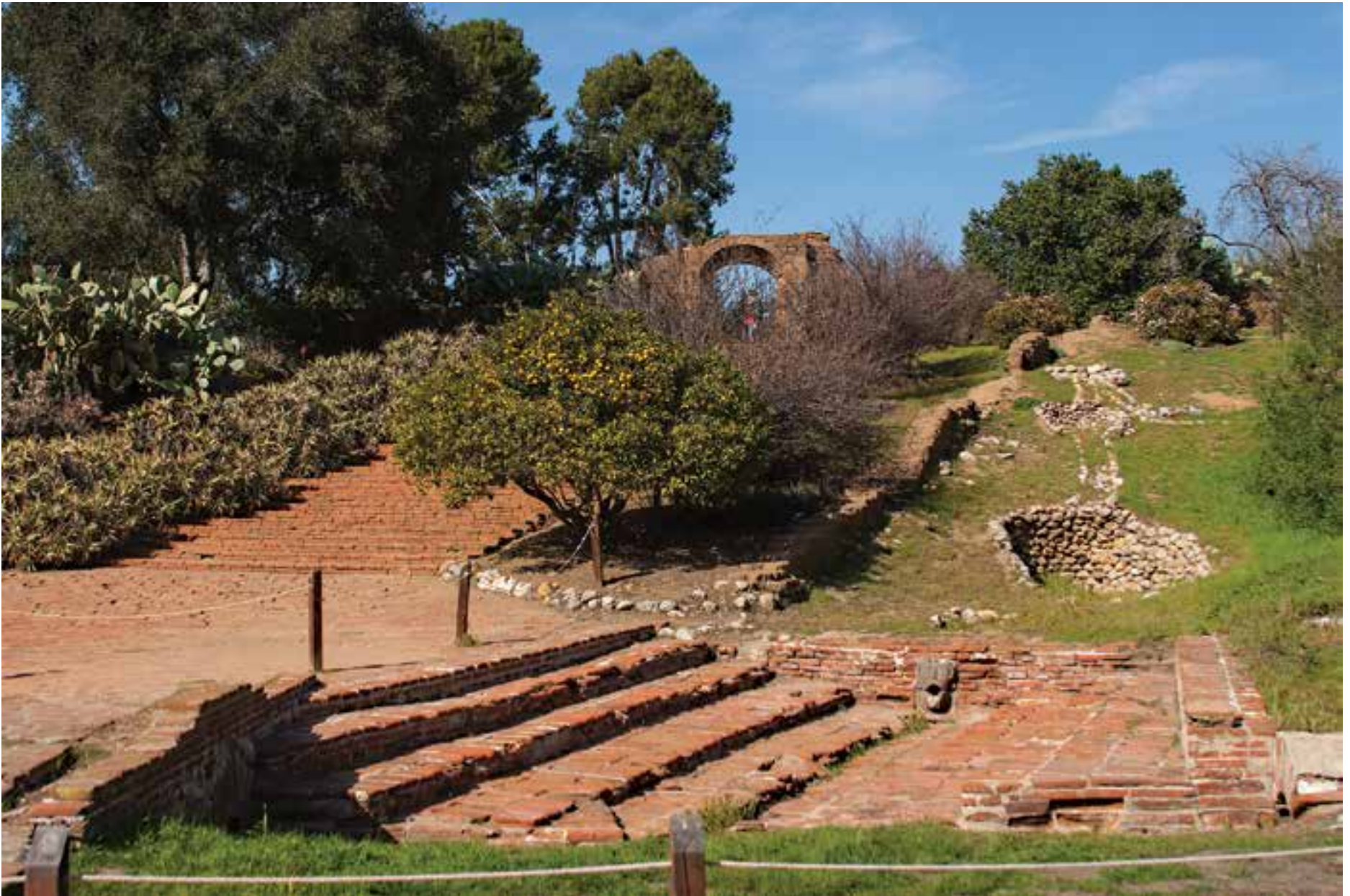
The lavanderia at Mission San Luis de Rey Francia is legendary, an original water source of the mission's using a charcoal filter, and rebuilt close to its original state during the later 20th Century.
