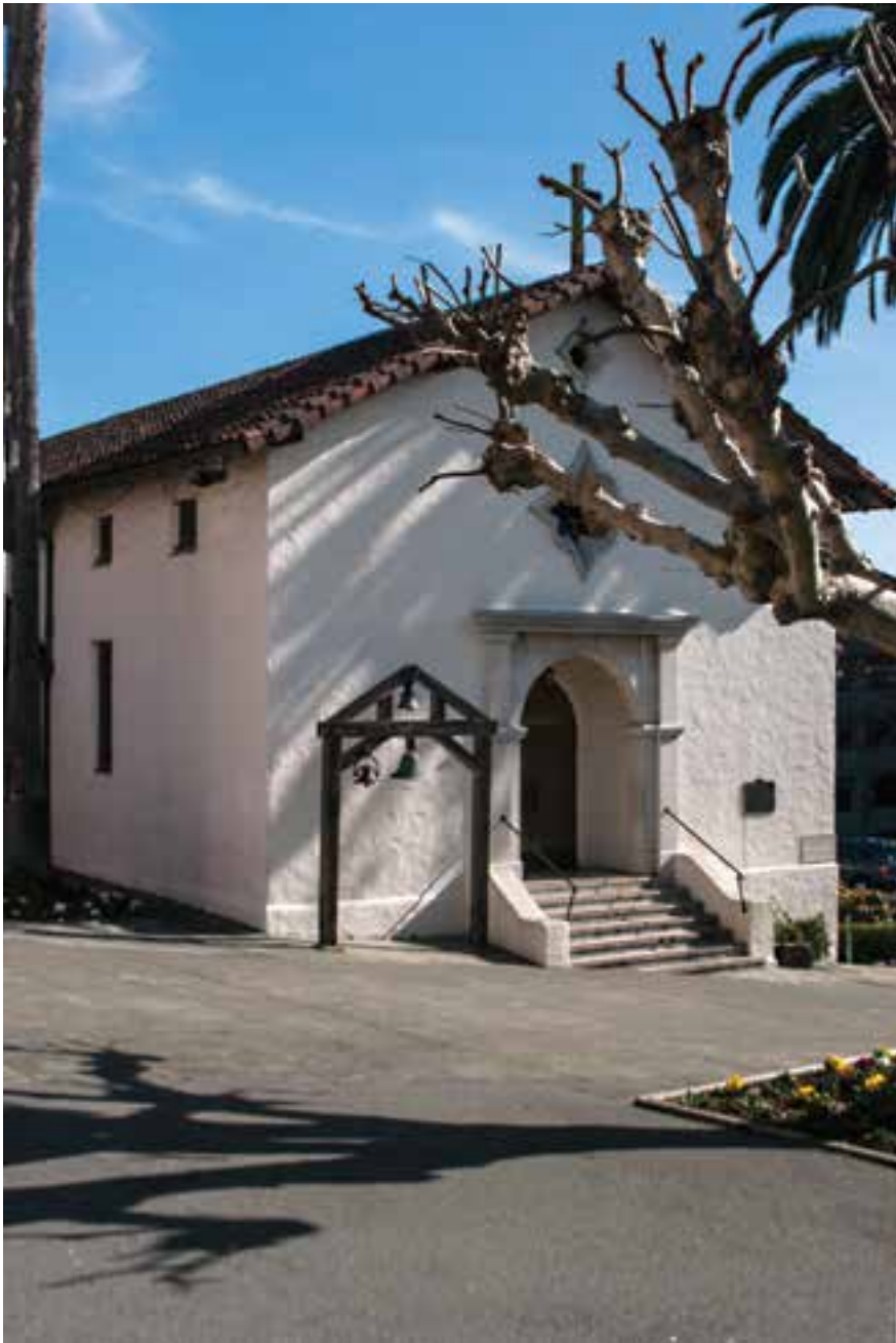
The Mission San Rafael Arcángel Chapel, displays the original bell scaffold.
