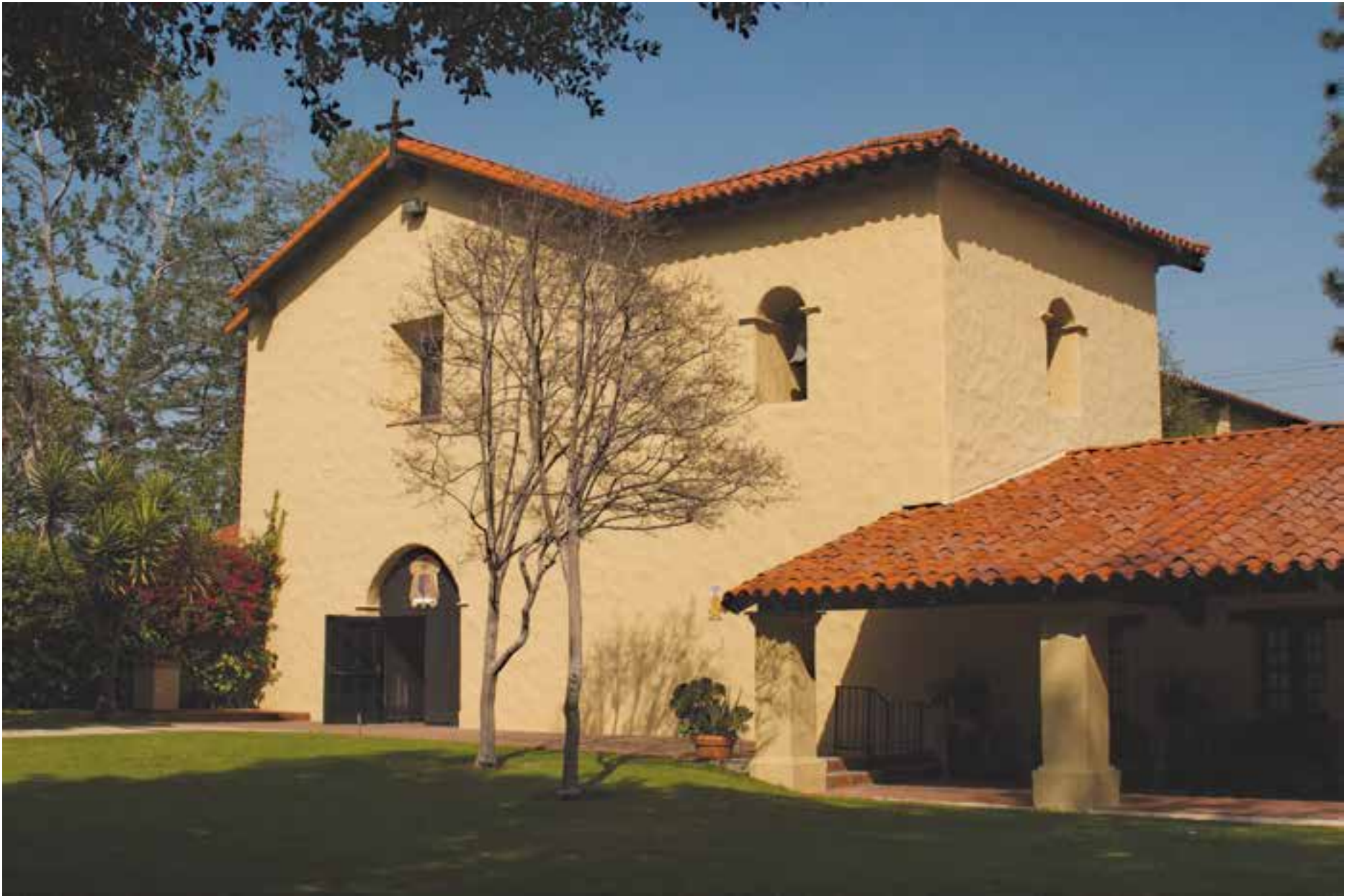
Mission San Fernando Rey de España church was completely leveled from a severe 1971 earthquake, then rebuilt over the next ten years. Nearby on El Camino Real, the “Long Building” two-story Adobe building, or Convento from the 1820s remained unaffected.
