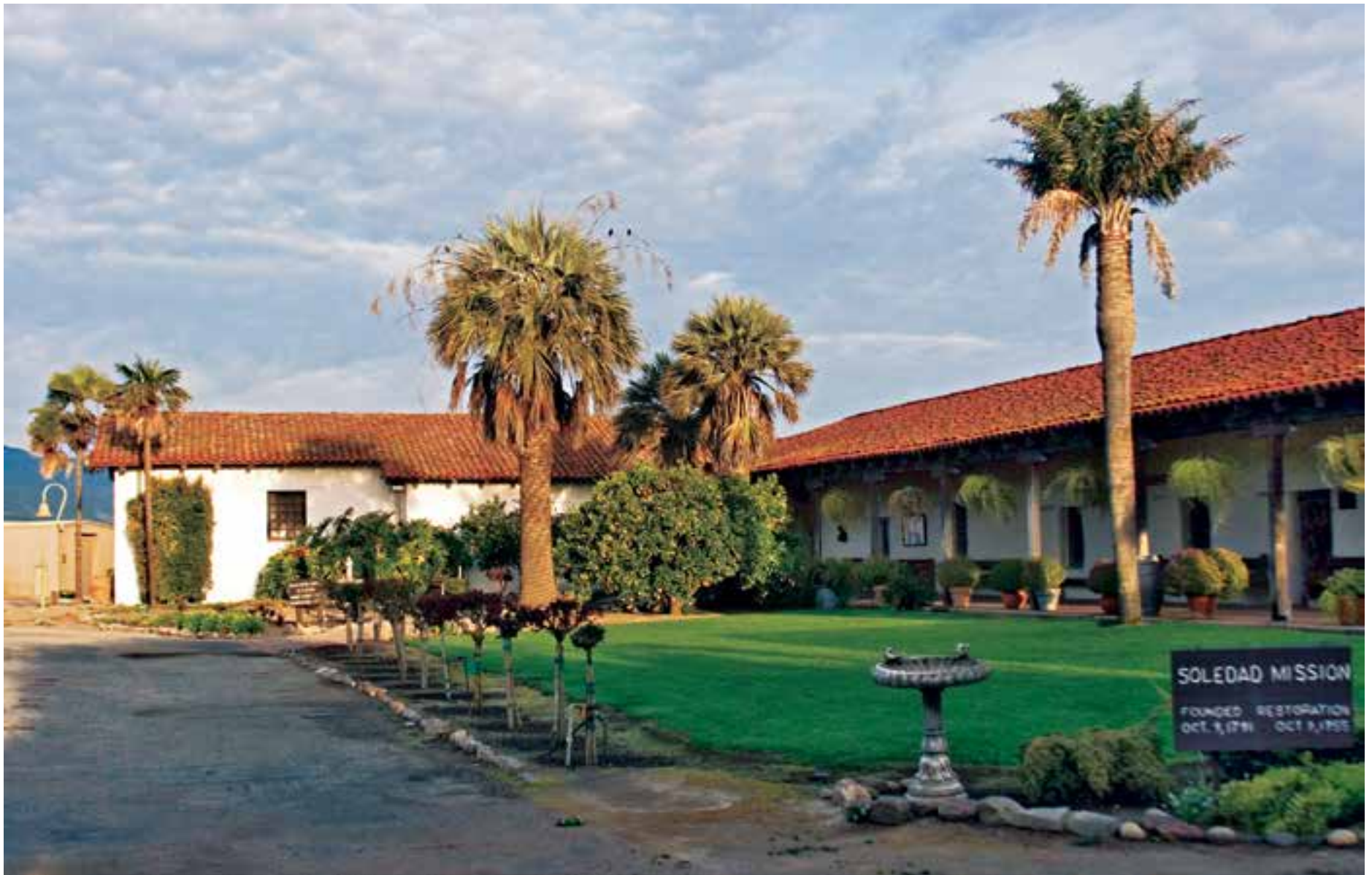
The Adobe Church and Convento are joined, and today in service and located in its original placid El Camino Real setting, near State Highway 101.
