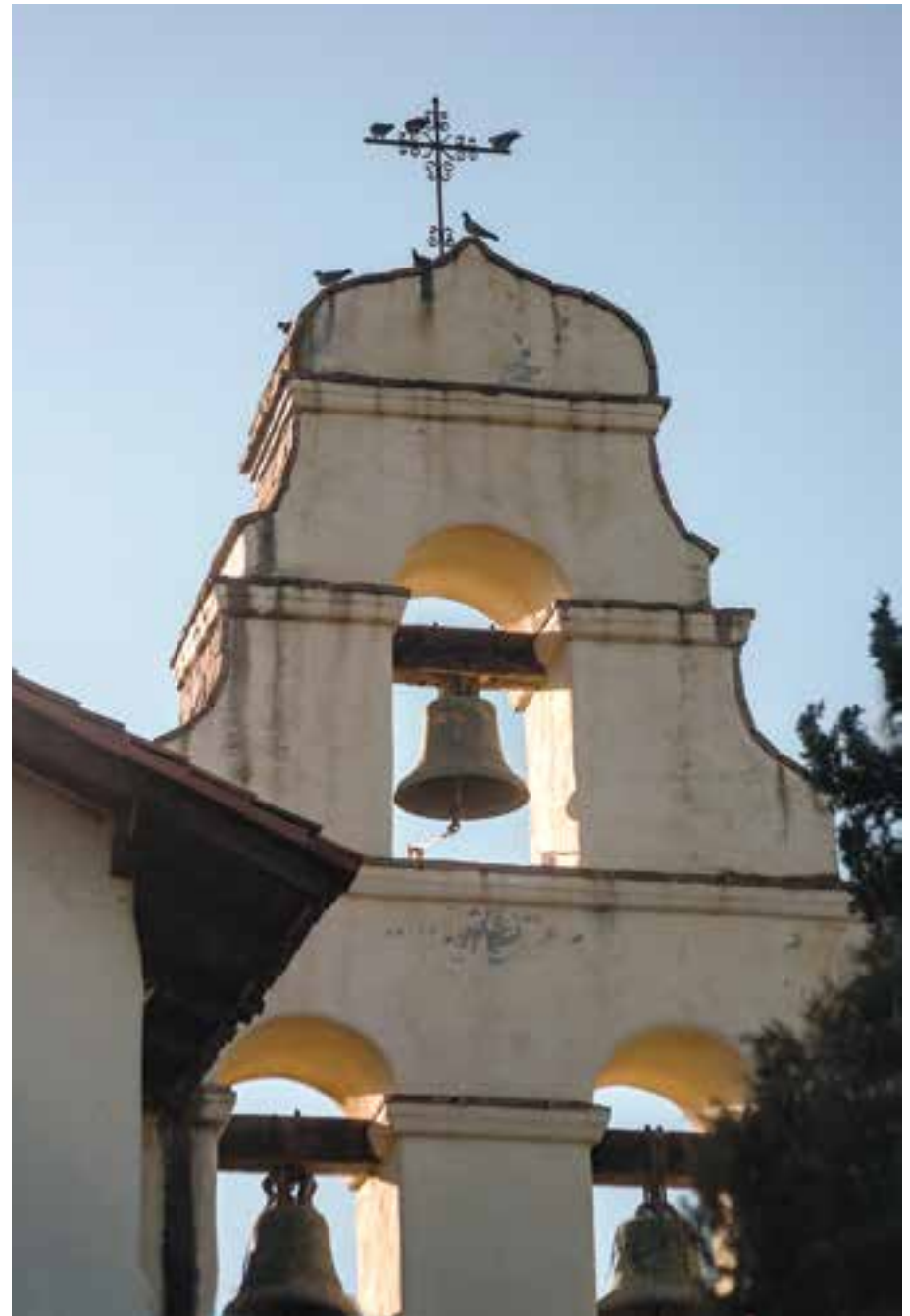
The Mission San Juan Bautista espadaña rises over the church wall, designed and built in the 20th century.
