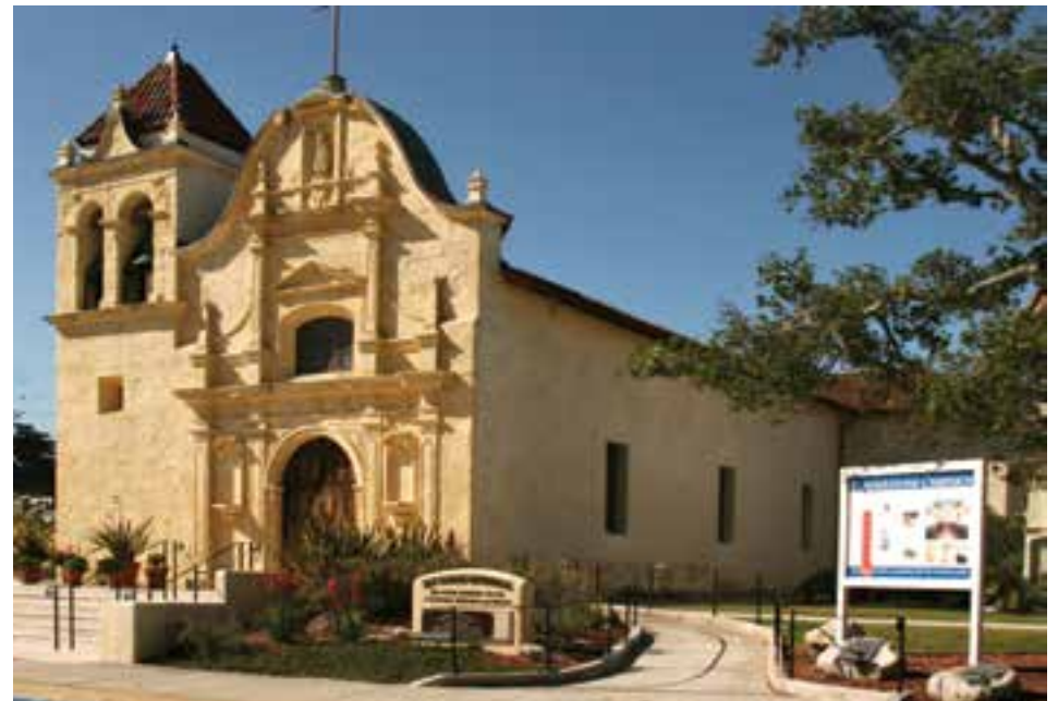
The San Carlos Presidio Chapel has been restored many times and currently retrofitted to comply with earthquake standards and refinished in a fresh traditional golden hue, often attributed to 18th Century royalty colors.
