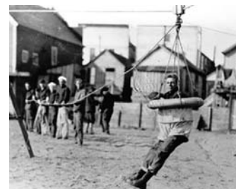
A breeches buoy, which would be carried out to a ship by pulleys, enabling sailors to step into the life ring and canvas sling to be rescued.
