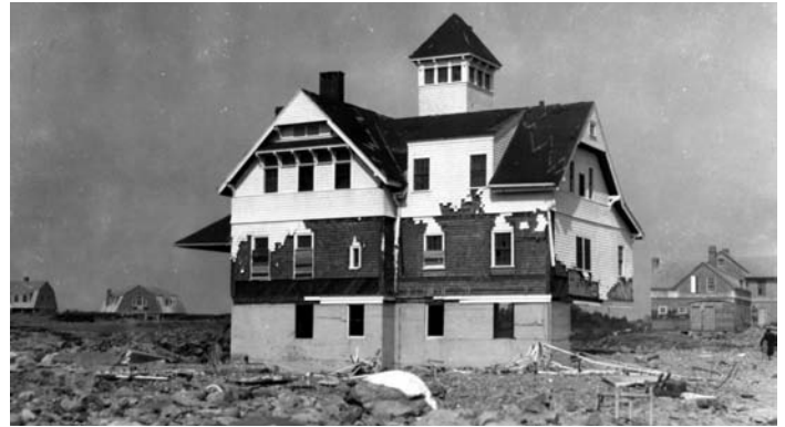
Storm damage to Boat Station Brenton Point due to the Great New England Hurricane. (U.S. Lifesaving Service Heritage Association)
