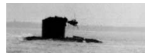
The remains of the lighthouse after the storm. After the storm's tidal waves struck the light, only the foundation remained. (U.S. Coast Guard)
