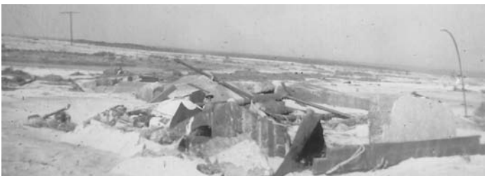
The remains of Station Moriches after the storm—just a foundation and sand. (U.S. Lifesaving Service Heritage Association)
