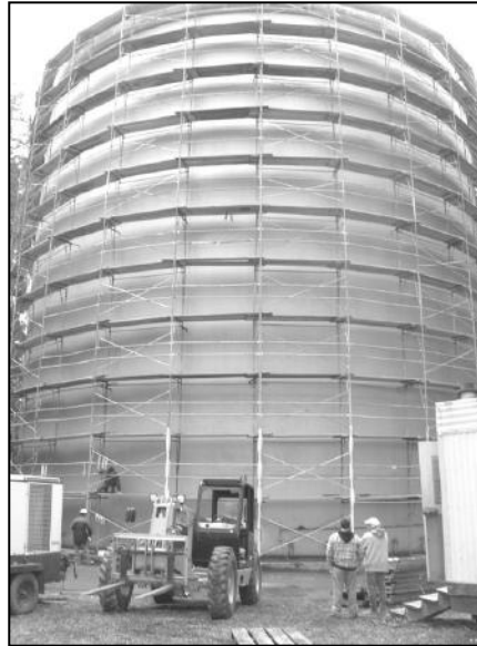
Canyon Park Tank During Recoating, 2005
