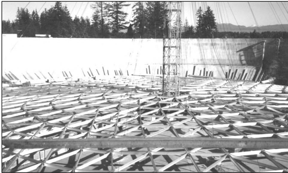
Crane Used to Hoist Roof Lattice Structure into Place, 2001
