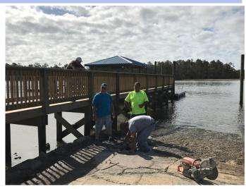
together all the loose concrete pieces that were a result of piling installation. Remaining are three or four more piling locations on the down slope of the boat ramp that need the same application of concrete. This can be accomplished with volunteers and approximately five cubic yards of material costing \$137.00 a yard. Therefore, it is recommended that the BOD consider approving up to \$1200.00 from the remaining pier funds. Or, utilize the annual budgeted \$1000.00 for pier repair.
