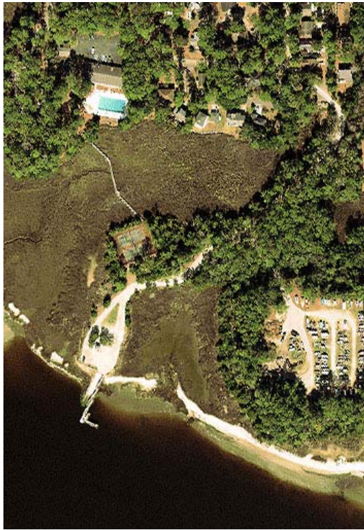
2014 aerial view of the waterway and Windjammer Village amenities - clubhouse, pool & playground area, tennis courts, marsh boardwalk, pier, and storage compound area.
