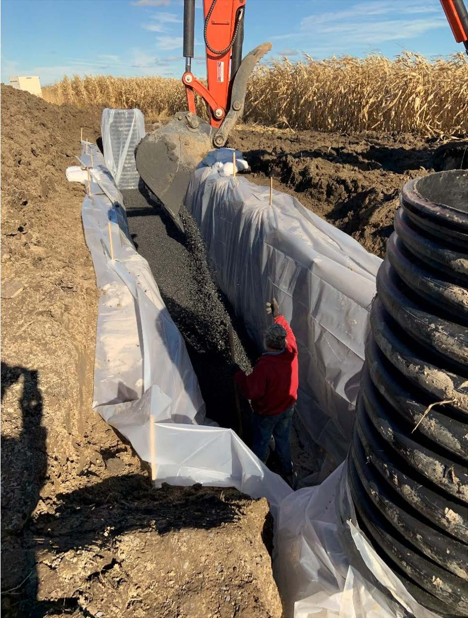
***Spreading and raking in activated alumina and iron***
