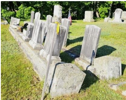
Pre photo of leaning stones, one row in danger of falling down over the other row if not fixed.
