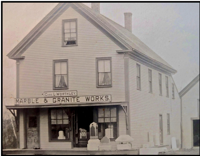
Charles Worthley's Marble and Granite company on Depot Street.
