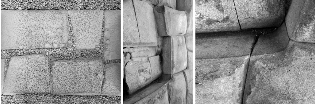
Fig. 3 A series of Inca constructions that reveal the voided wedge between stones
