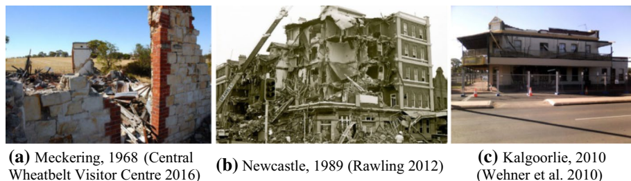
Fig. 1 Damage of masonry structures in earthquakes
