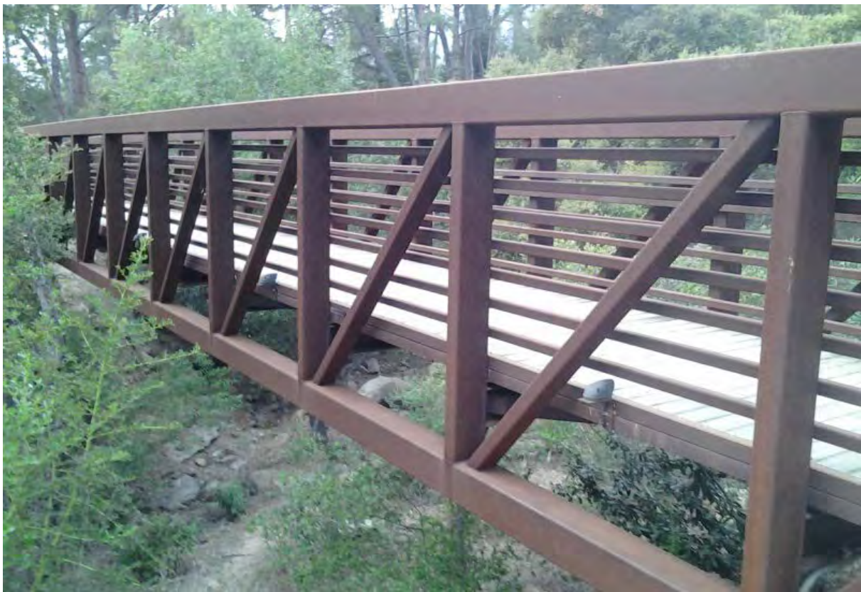
Westmont College Ped Bridge (129' span, 7' truss height)
