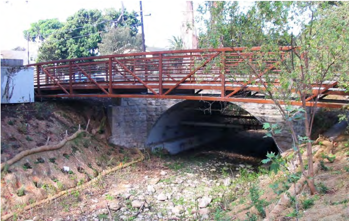
Mason St Ped Bridge
