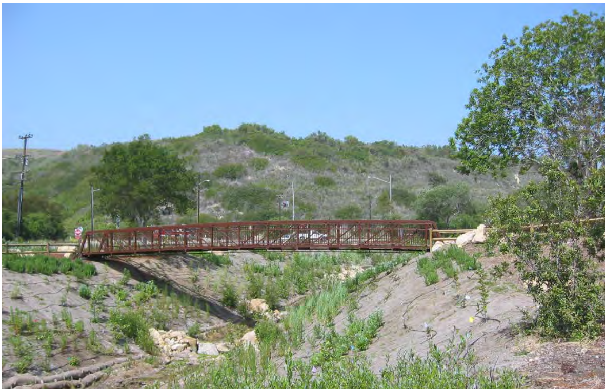
Arroyo Burro Ped Bridge (72' span, 4'3" truss, 5'6 width, vertical pickets)
