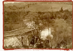
Historic stone bridge over Mission Creek in the 1890s, looking northwest. Photo courtesy Gledhill Library, Santa Barbara Historical Museum.
