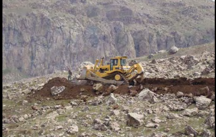
Line clearing for 2D dynamite acquisition
