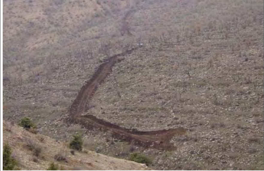
Line clearing for 2D dynamite acquisition
