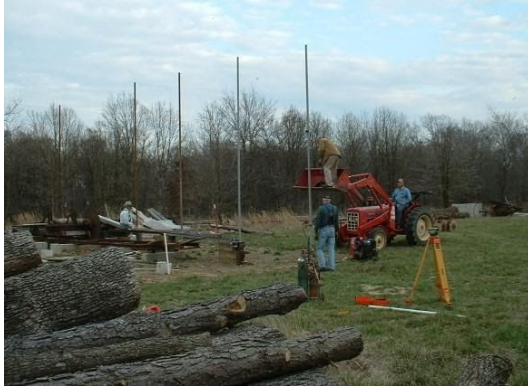
Building the Sawmill Shed at Tired Iron March 7, 2005
