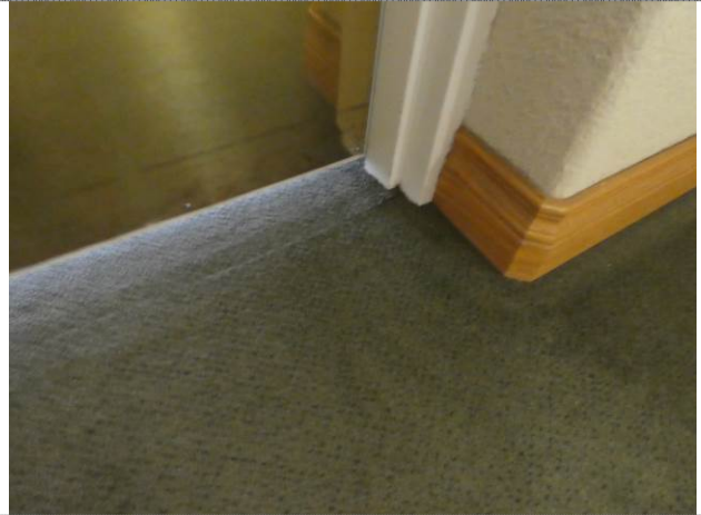
Lifting seam in carpet
