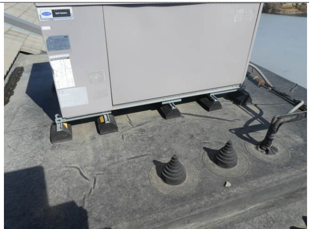
SBS roofing under mechanical
