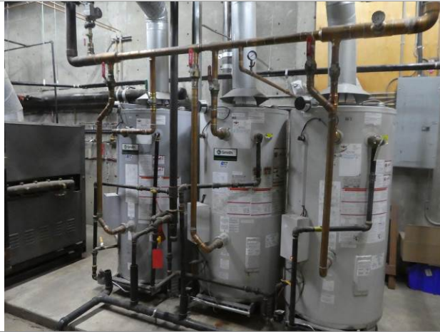
A.O. Smith hot water heaters/tanks - 100 gal M: BTRC400A118 S: 1527M00217, 1220M001330 & 1408M001824
