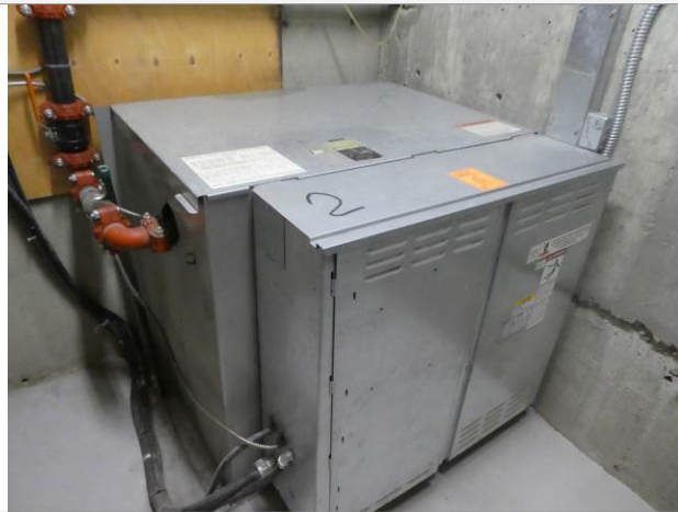
Elevator hydraulics
