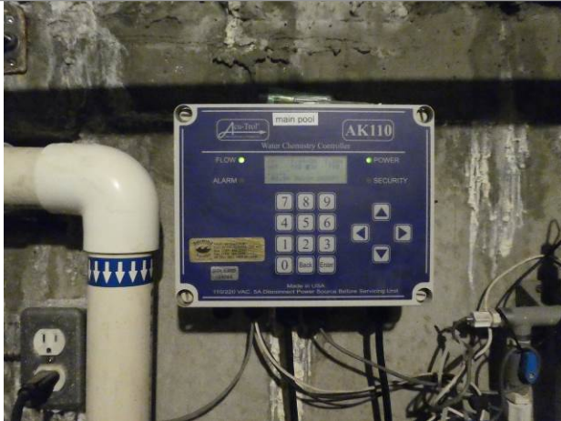
Water chemistry controller
