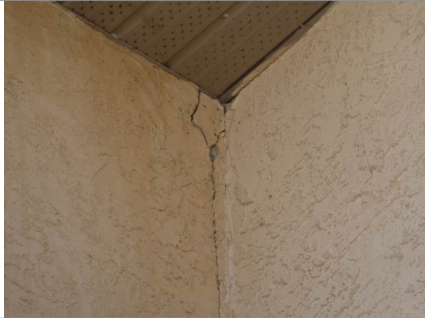
Damaged stucco at interior corner
