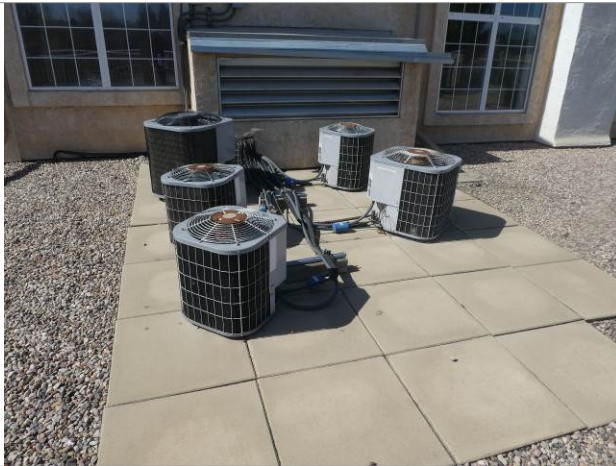
Rooftop A/C unit - Carrier M: 38AK5014 - 120 S:4902F92298
