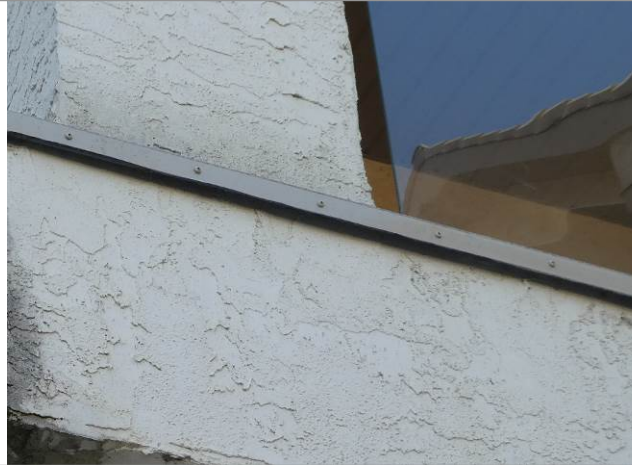
Clamping bar installed at drip edge
