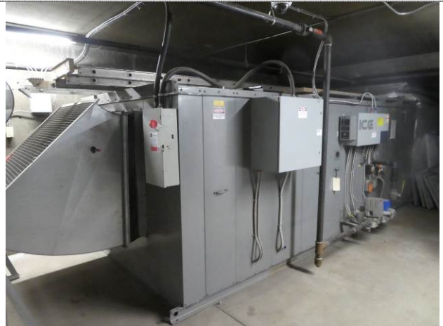
Ice makeup air unit M: BMA136XDA S: 27945B0209
