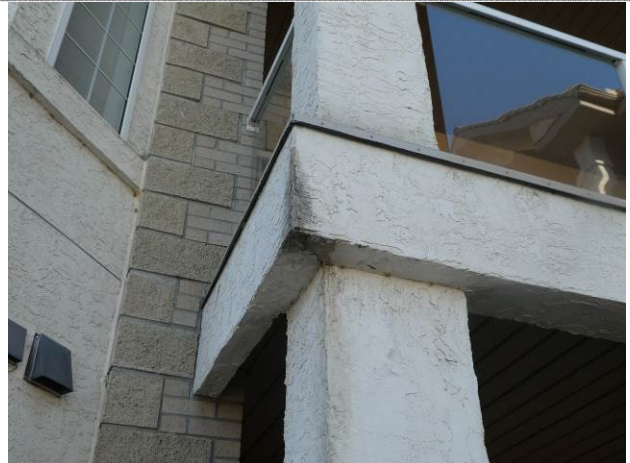
Stained stucco on balcony fascia – indicative of poor water drainage
