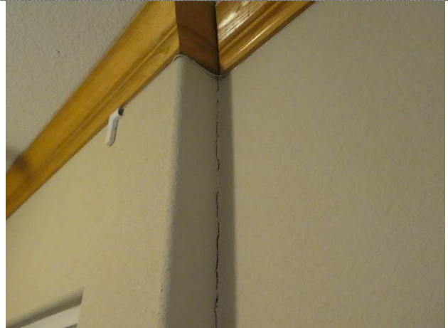
Cracking in wall finish
