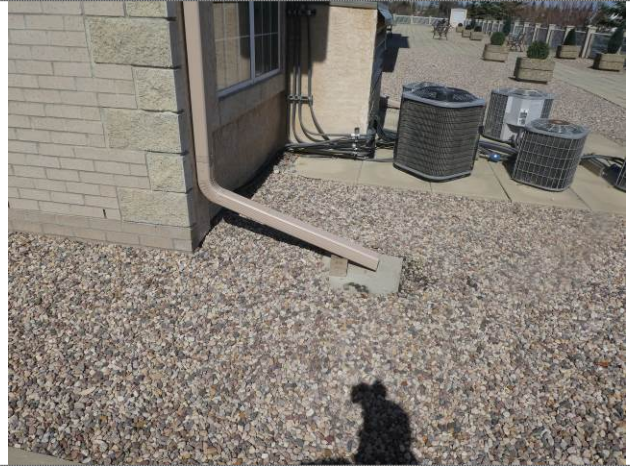
Typical downspout termination
