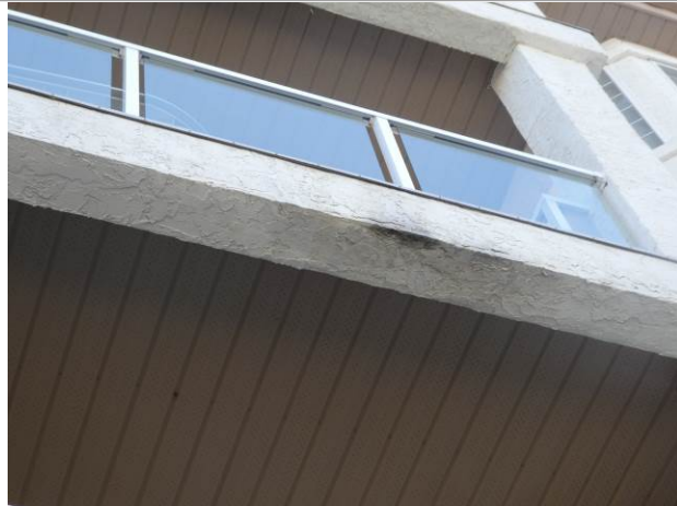
Stained stucco on balcony fascia – indicative of poor water drainage
