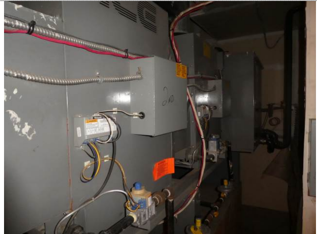
Hallway makeup air unit - Ice M: UPB 12-800 AGR S:27945A0209
