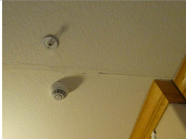
Cracking in ceiling finish
