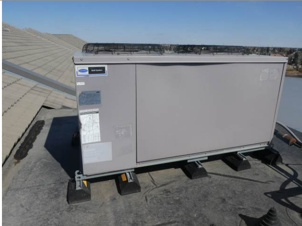
Rooftop A/C unit - Carrier M: 38AK5014 - 120 S:4902F92298
