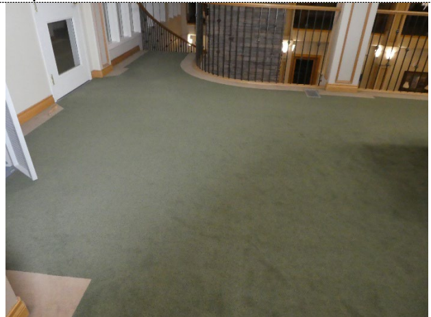
Amenities room (2 nd floor) carpet
