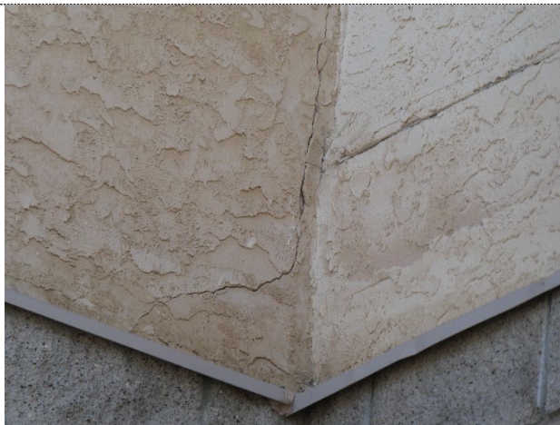
Cracked stucco
