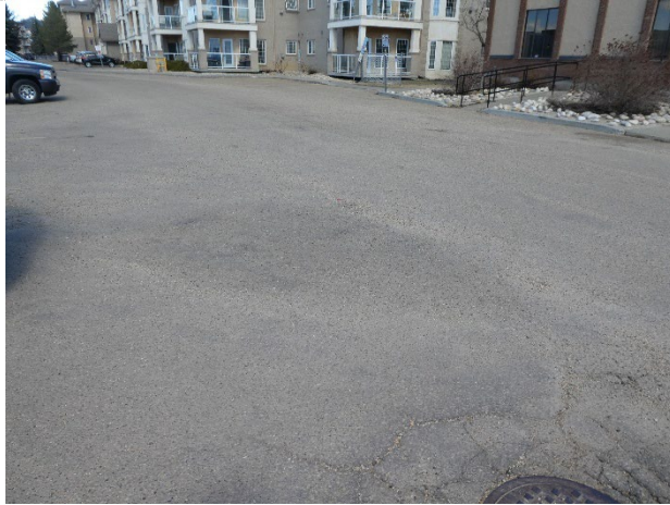
Asphalt parking & roadways
