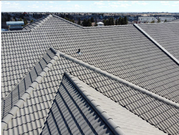
Concrete roof tiles
