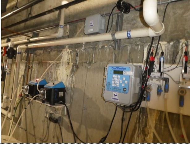
Peristaltic pumps & water chemistry
