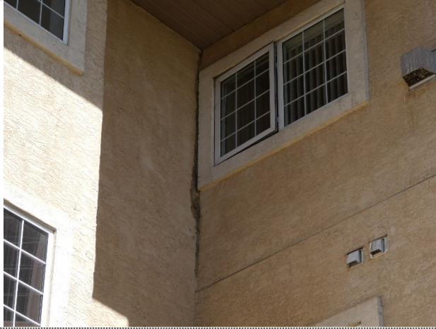
Cracked/damaged stucco
