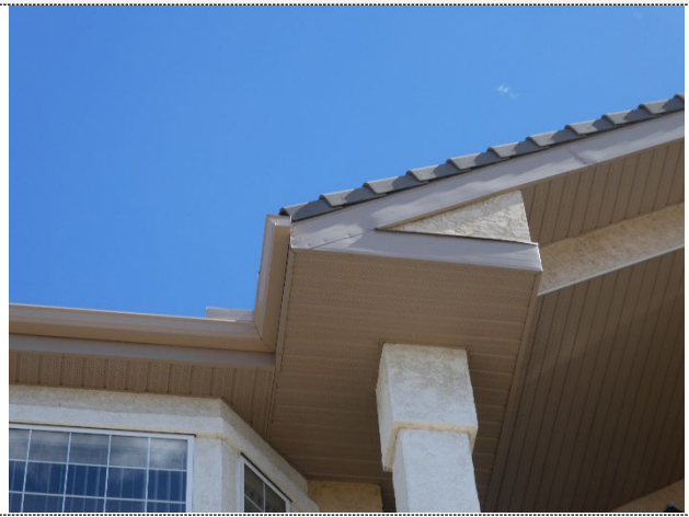
Fascia & soffit at roof overhang
