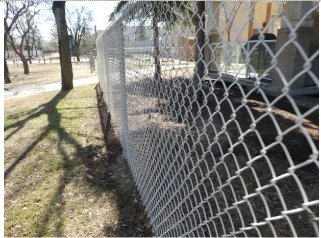
Chain link fencing
