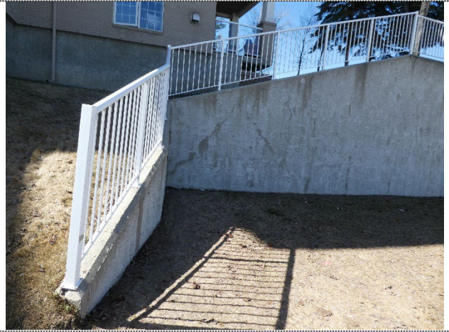
Railings & retaining wall – north
