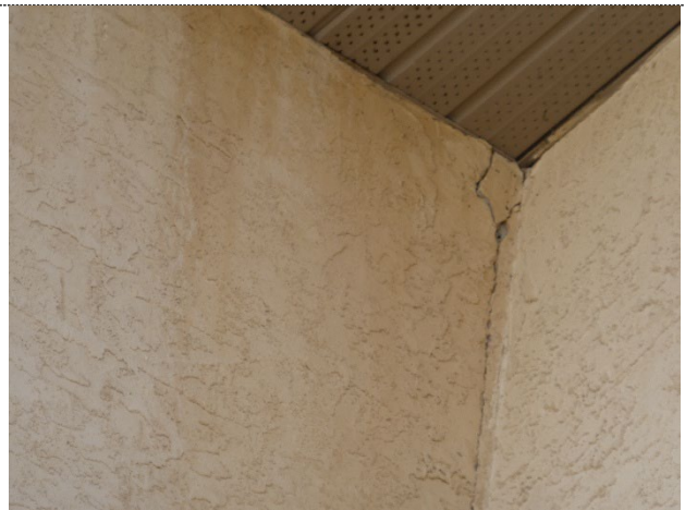
Cracked stucco
