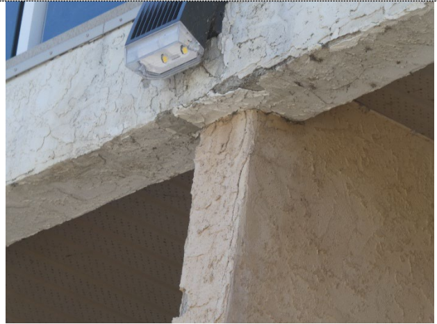
Deteriorated stucco on balcony fascia
