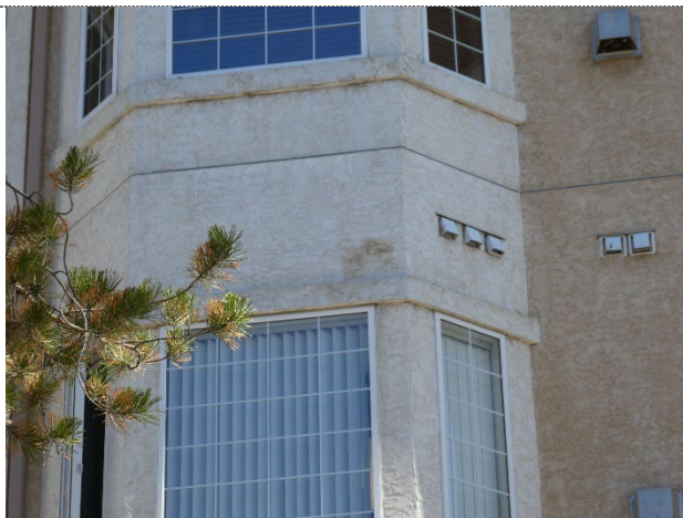
Deteriorated stucco – architectural reveals
