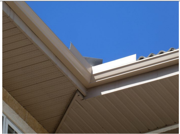
Flashing installed at inside corner
