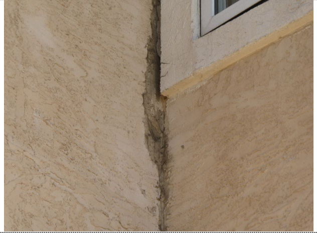
Cracked/damaged stucco
