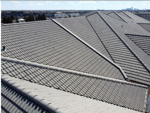
Concrete roof tiles
