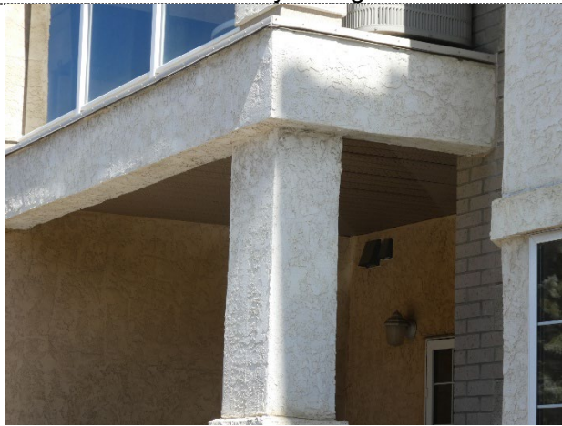
Balcony fascia & post cladding
