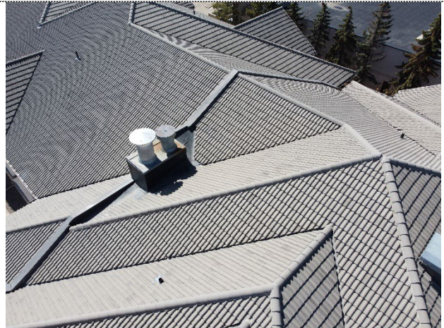
Concrete roof tiles
