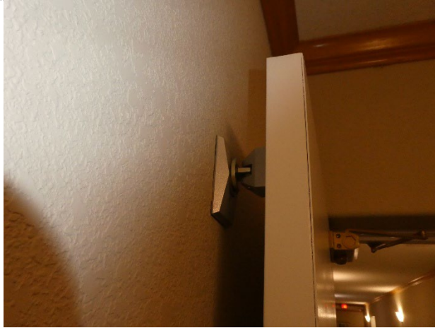
Fire release mechanism
