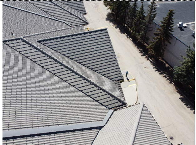
Concrete roof tiles
