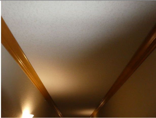
Ceiling paint finish in hallway
