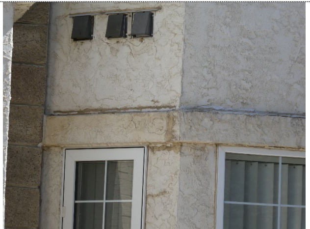
Damaged stucco
