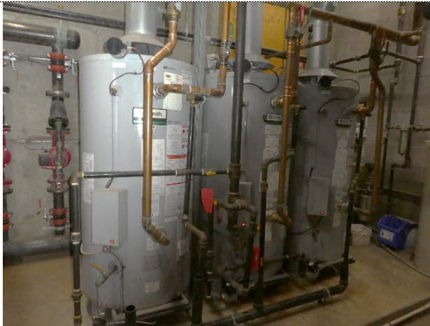
A.O.Smith hot water heaters – 100 Gal M: BTRC400A 118 S: 9281001006 & 2547146128596 & 2609147289744
