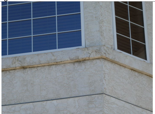
Deteriorated stucco – architectural reveals
