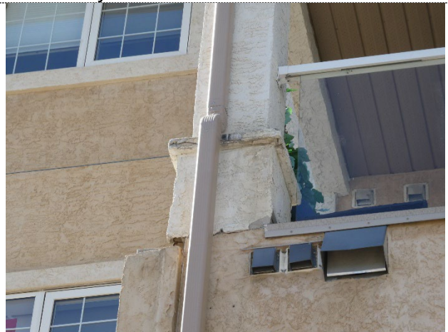
Deteriorated stucco
