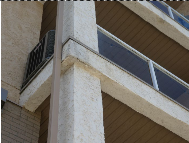
Deteriorated stucco on balcony fascia
