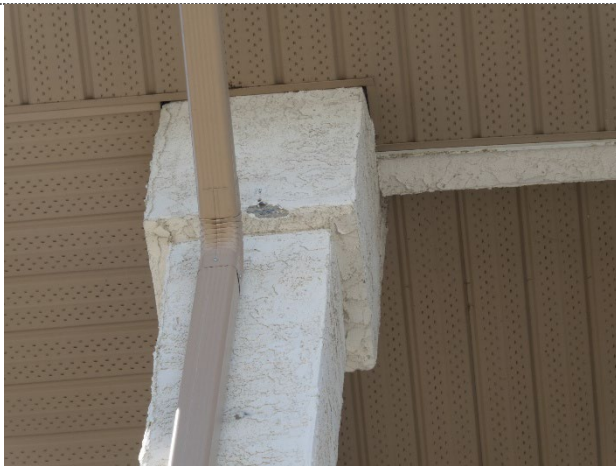
Deteriorated stucco
