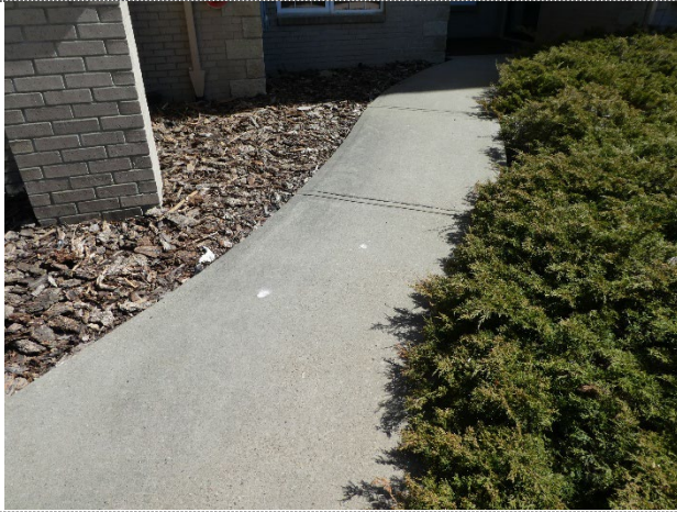
Walkway in fair condition
