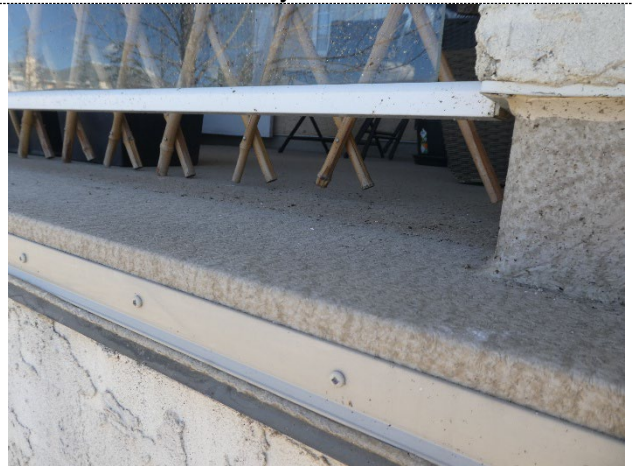
Clamping bar installation on balcony membrane
