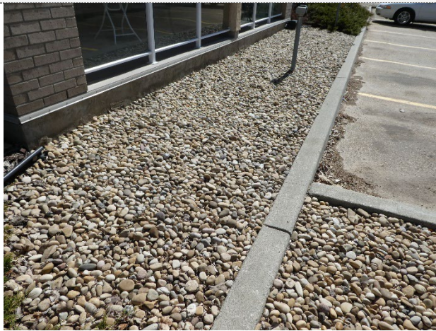
Stone installed at front of building
